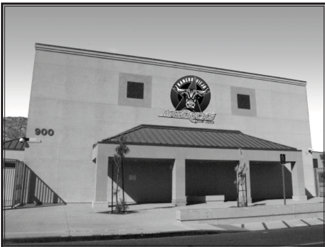
Rancho Viejo Middle School Administration Building
